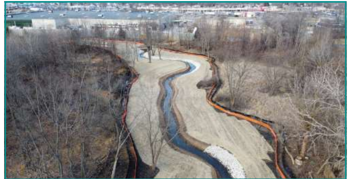
East Branch Tributary 2 Channel Maintenance Project
