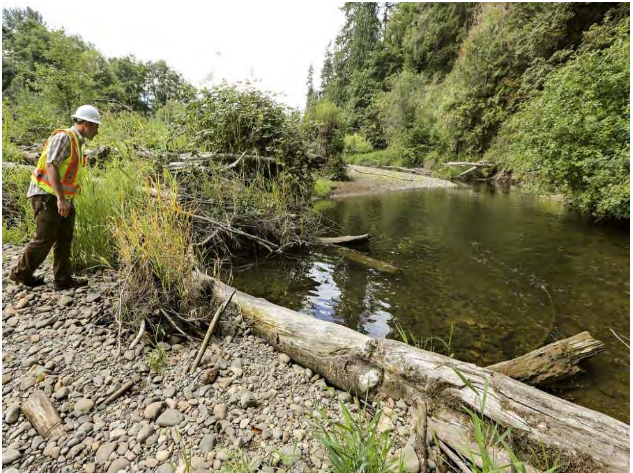
Figure 13. Bank large wood structure, Cowlitz River, Washington. Five years after construction.
