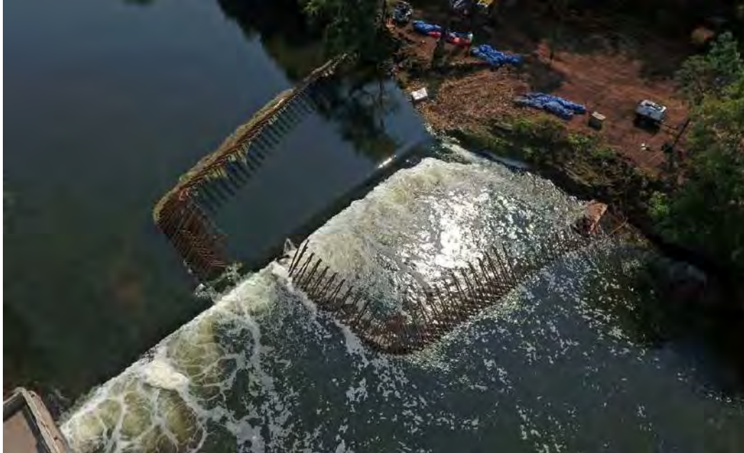
Plate 2. Dewatered East Side of River Before Removal of Structure (Photo Credit: FPDWC)
