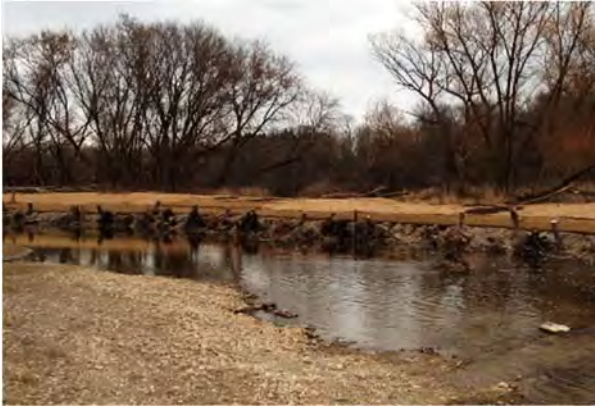
Figure 12. Large wood crib structures, Sheboygan River, Wisconsin. During (left) and two years after construction (right).
