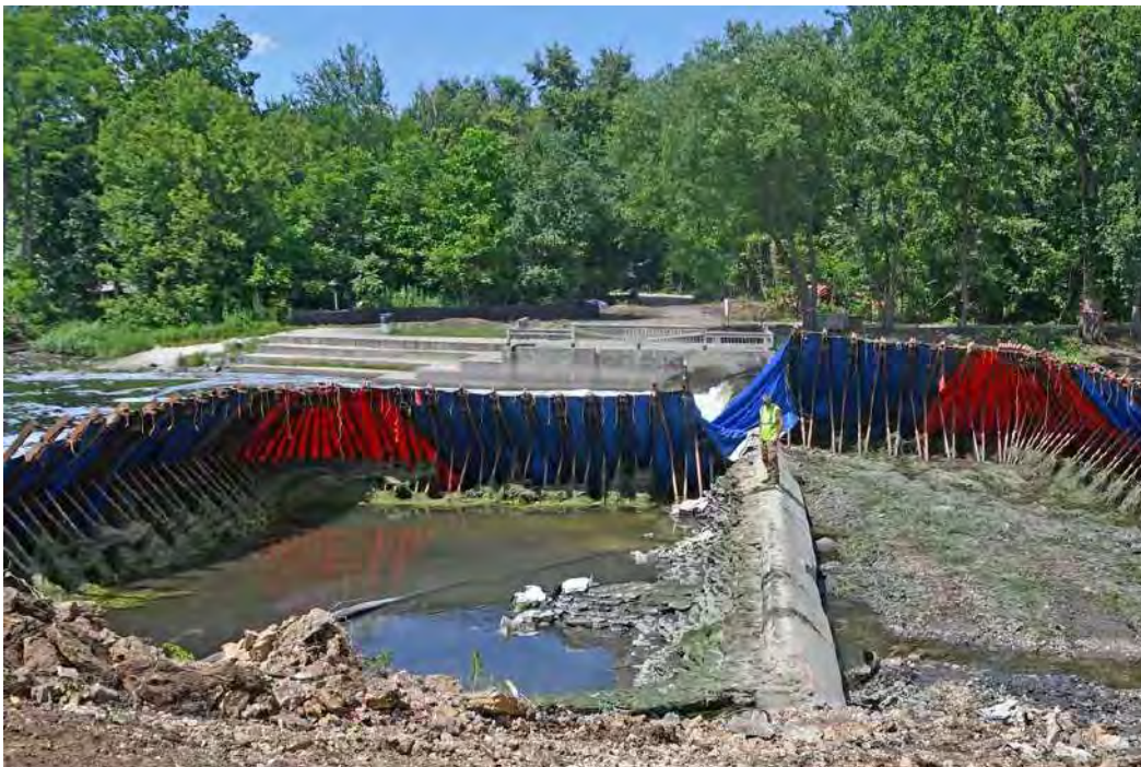
Plate 2. Dewatered East Side of River Before Removal of Structure (Photo Credit: FPDWC)
